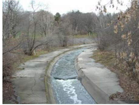
Yonge York Mills Flood Channel
